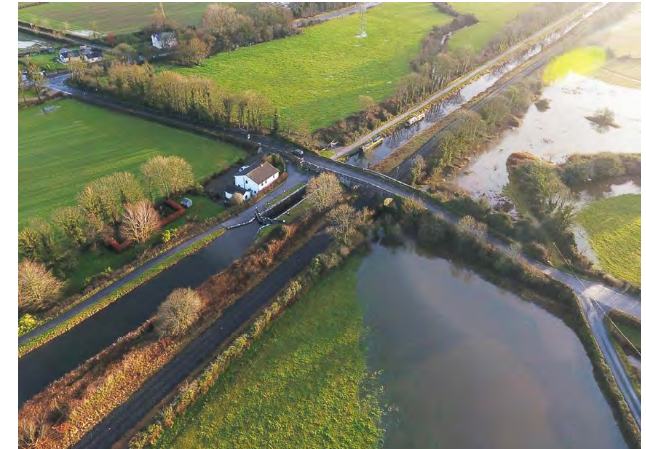
View of flooding at Jackson's Bridge – February 2021
