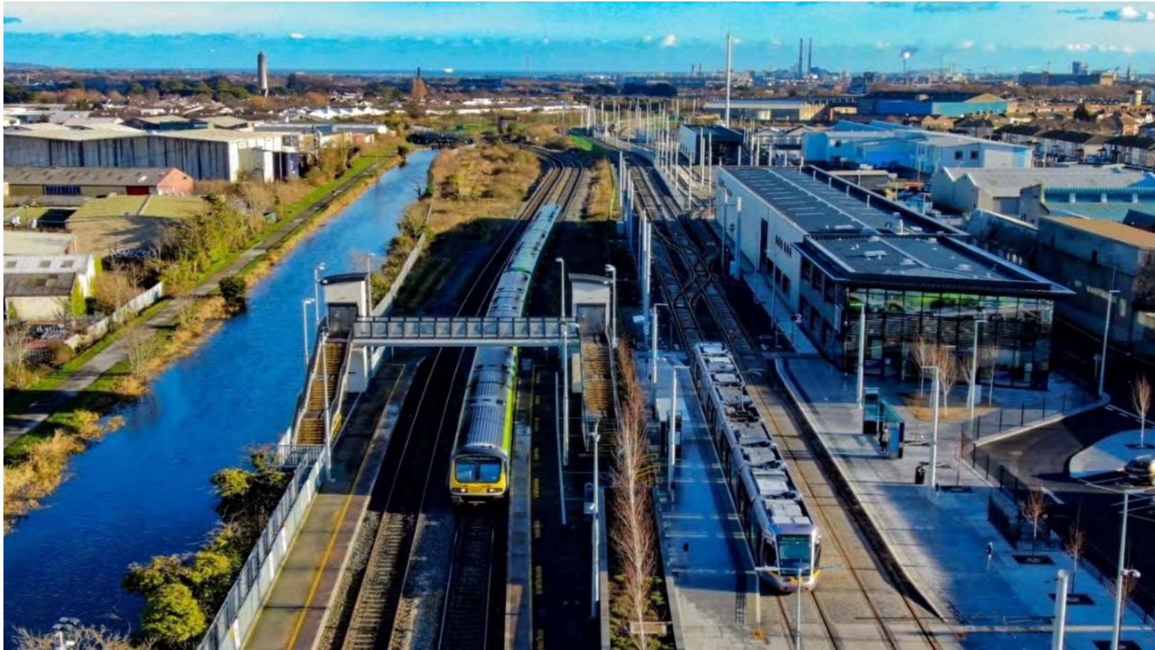
Aerial view Broombridge integrated rail and LUAS stations
