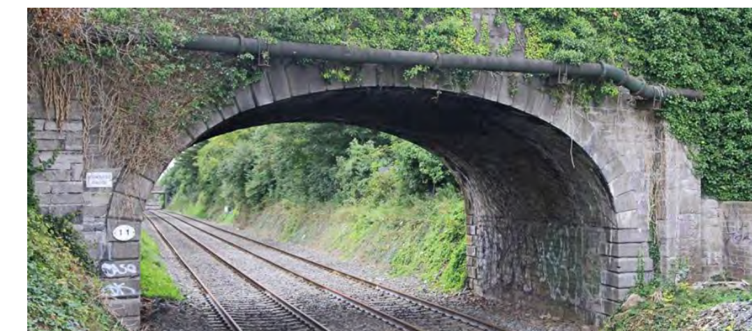
View of Castleknock Road railway bridge
