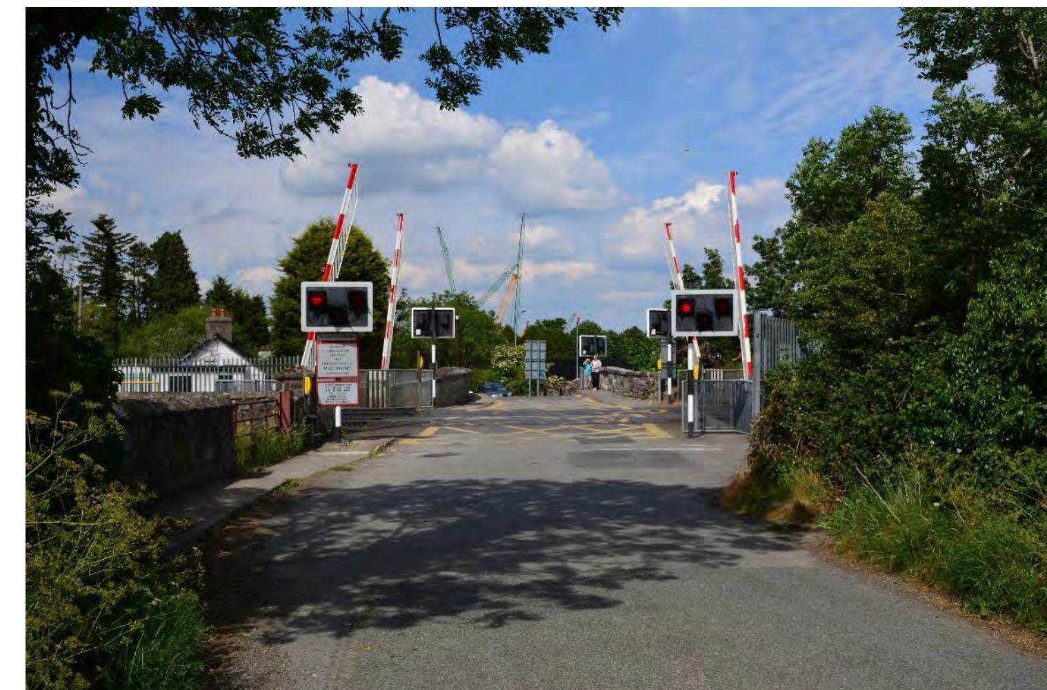
View of Blakestown level crossing
