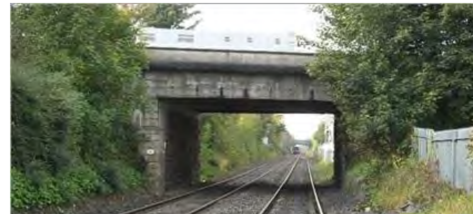
View of old Navan Road Bridge
